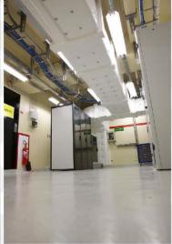
NuDUCT 5190 is a flexible protection, providing up to 2 hours of fire protection depending on the configuration. It is adaptable to the environment. This protection consists of mineral wool, refractory glue and a protective fabric.
