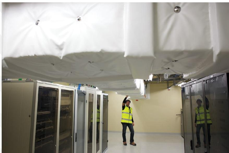
NuDUCT 5110 is a flexible protection, ensuring protection up to 2 hours, depending on the configuration. It is adaptable to the environment. This protection is composed of mineral wool, glue refractory and a protection fabric. This complex has a thickness of 80 mm.
